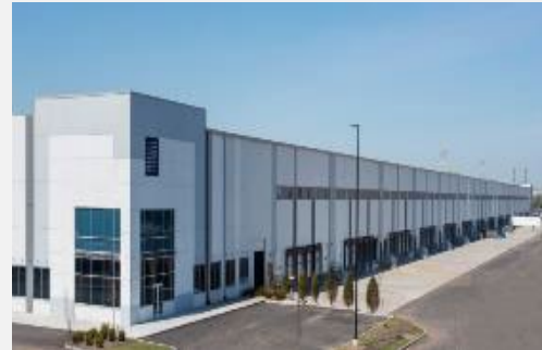
586 Gulf Avenue, Staten Island, NY
