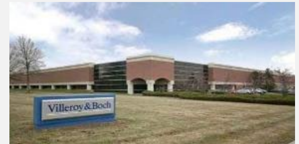
3 South Middlesex Avenue, Monroe, NJ
